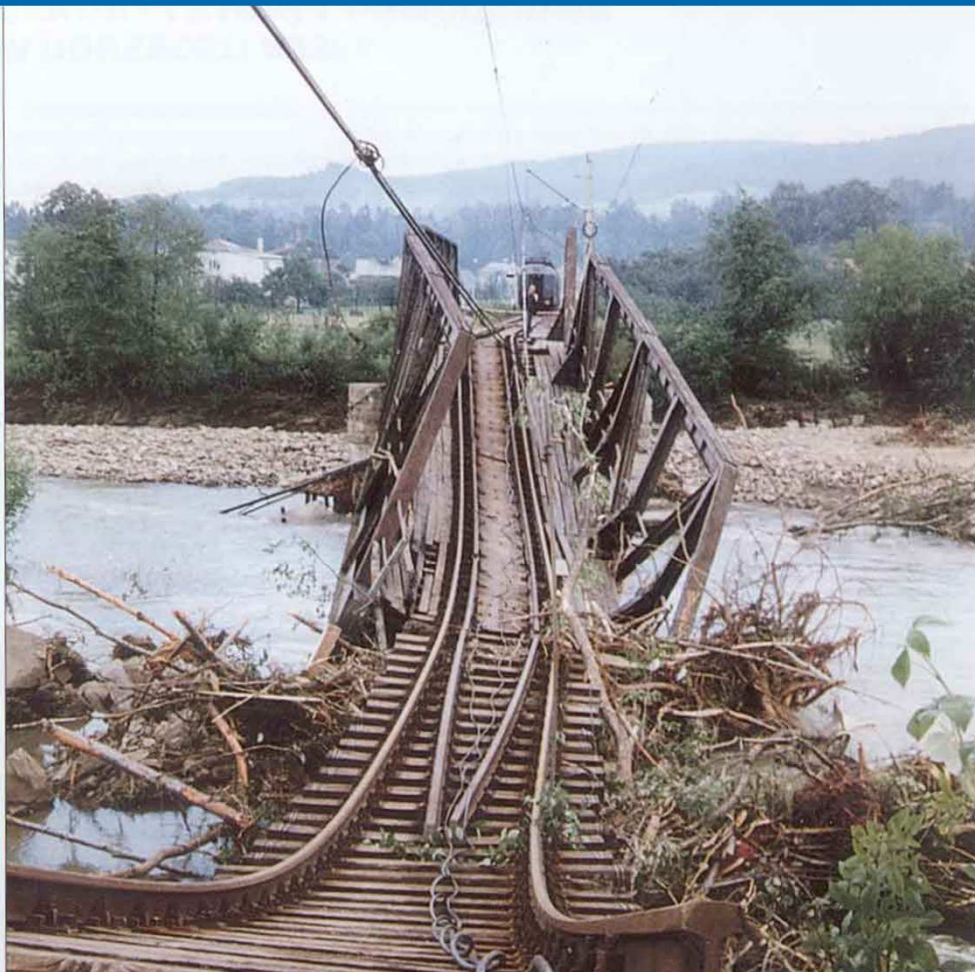
Flood damage in the Oder River basin, July 1997 (Courtesy IIHR)
