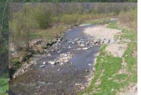
4.3 – When designing and building rapid hydraulic structures one has to bear in mind many construction and exploitation problems stones on the RHS apron slope plate, scouring problems downstream of the RHS, influence of RHS on upstream part of the channel and a sill situated at the crest part of the RHS
