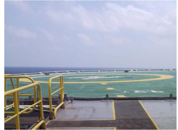
ISW- tilted helipad (AFTER appropriate action) Previous displacement 189m, broken drill string
