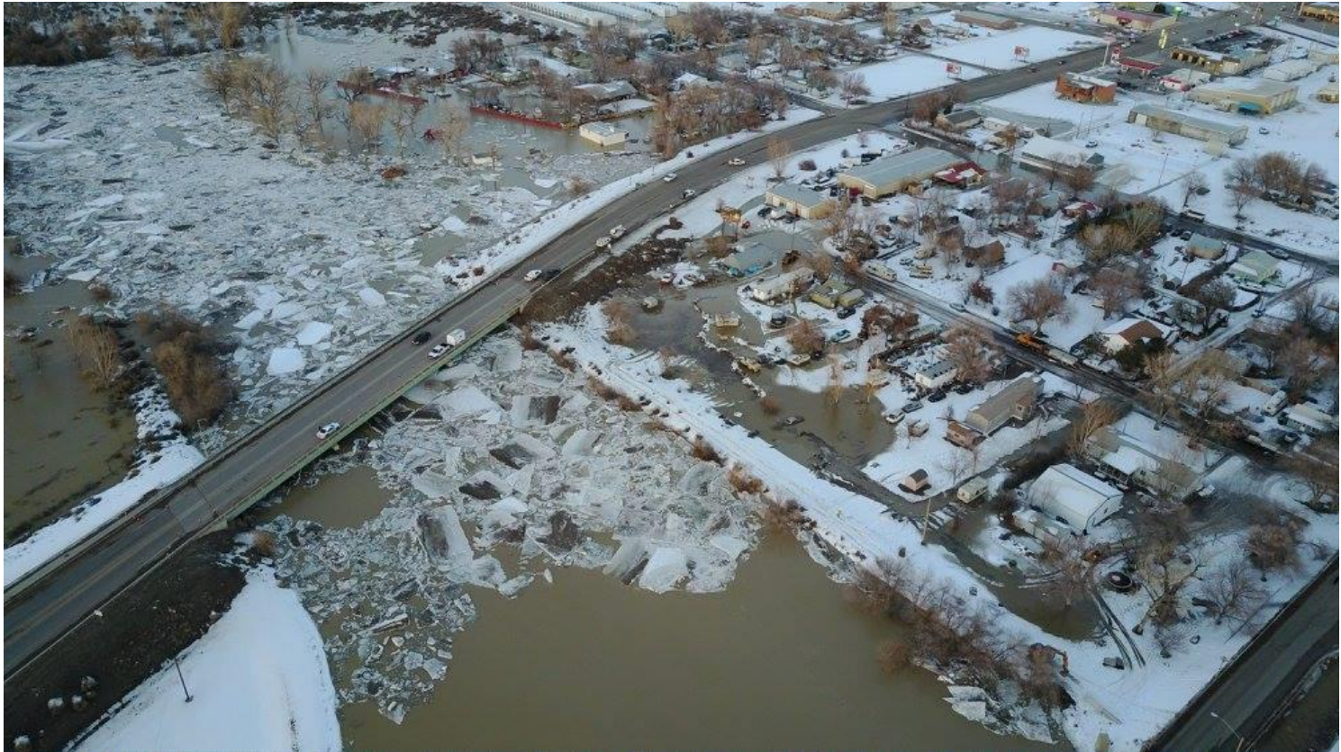
Ice blockage at a bridge forms jam on the Bighorn River, Wyoming
