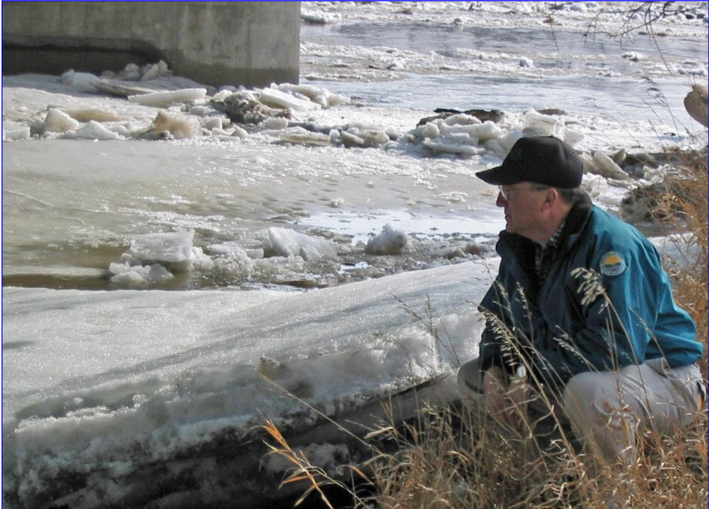
Ice on Union Dike, Platte River, NE
