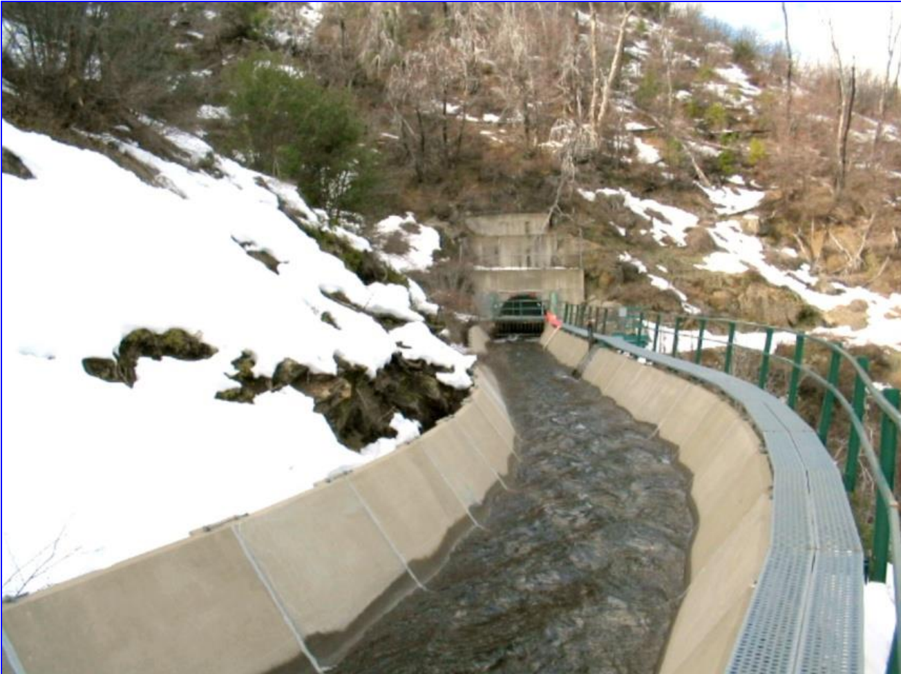
El Dorado Water Diversion System, Sierra Nevada Mountains, CA-NV
